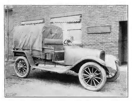
LIGHT REPAIR TRUCK ON DODGE CHASSIS. Special body with tools for making minor motor repairs.
