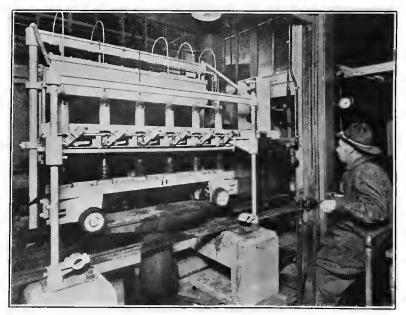
MACHINE FILLING 75-MILLIMETER SHELL WITH MUSTARD GAS.
