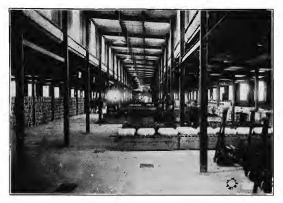
SHELL DUMP AT EDGEWOOD ARSENAL. This picture shows filled shell being stored for leakage test before being painted.
