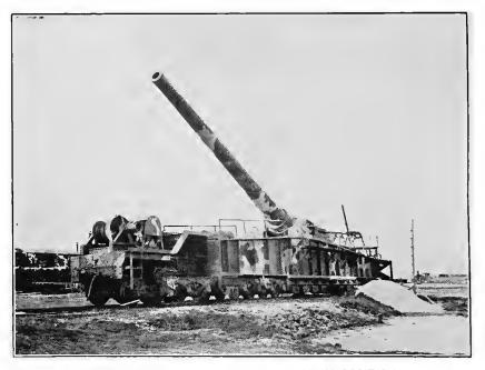
12-INCH RIFLE ELEVATED TO ITS MAXIMUM POSITION. It is capable of hurling a 700-pound shell 25 miles. This is a modified Schneider type of carriage.
